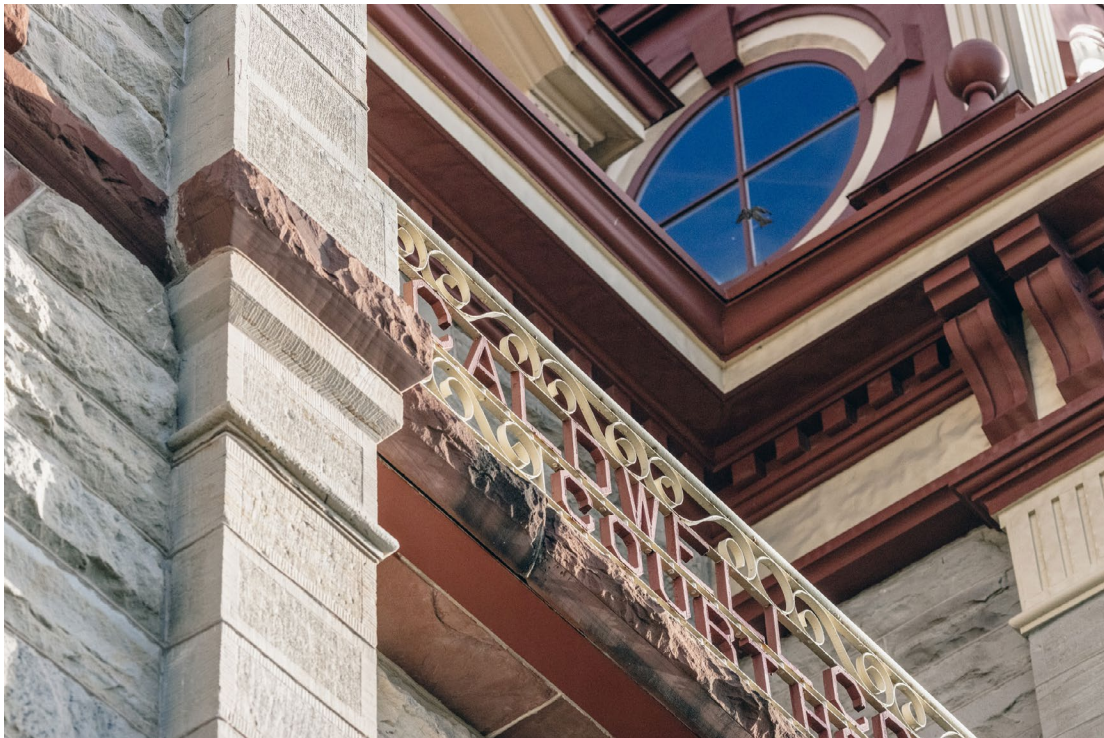
Caldwell County Courthouse, Lockhart, Texas.
